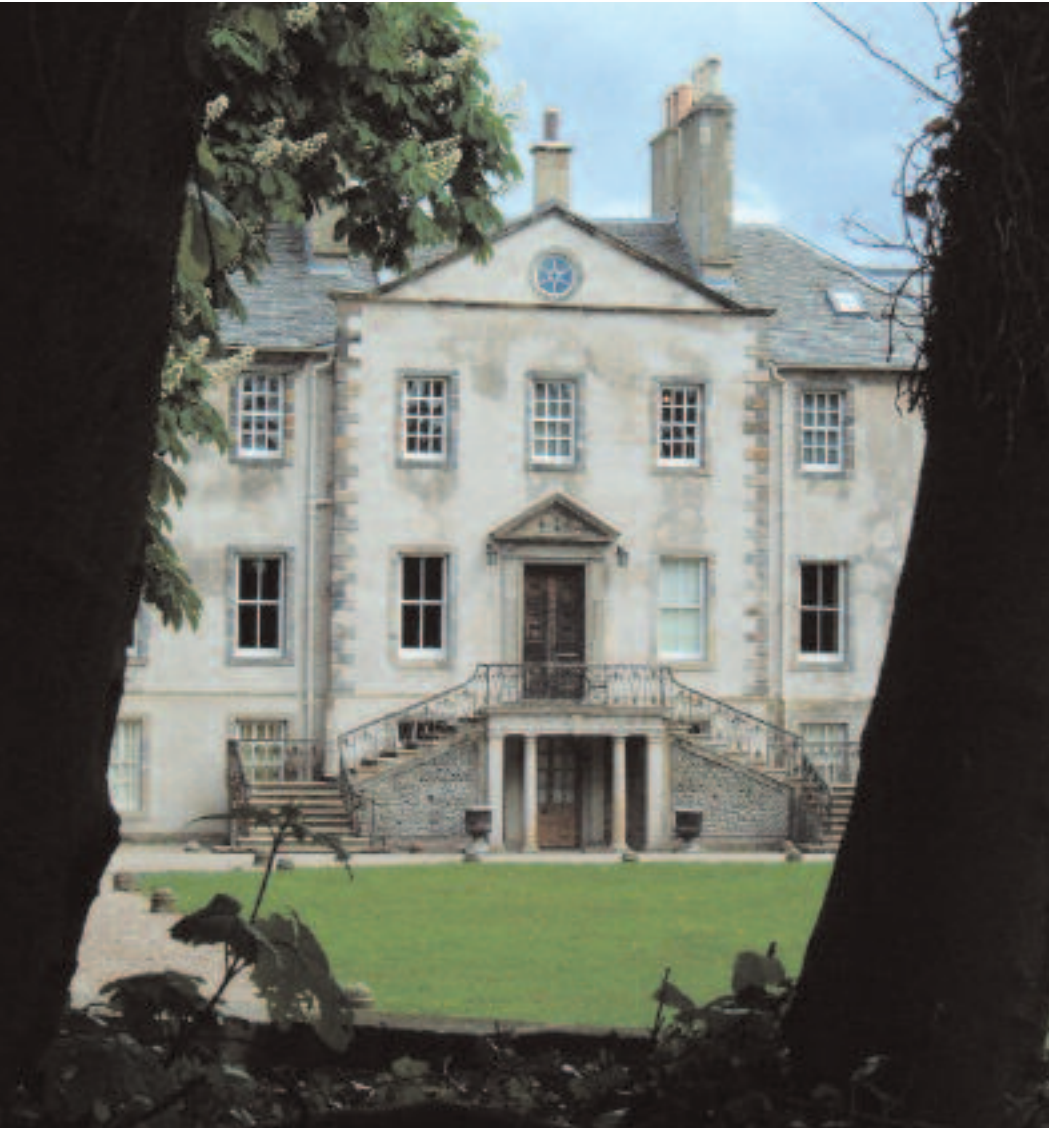
Newhailes House, Musselburgh, LDN Architects. © National Trust for Scotland
